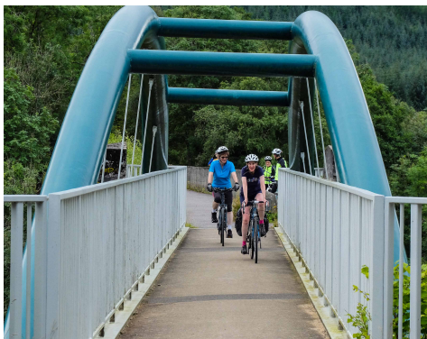
New Viaduct at Strathyre
